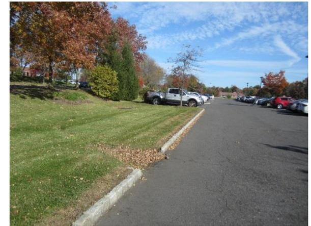
Rows of parking spaces can be replaced with pervious pavement to capture and infiltrate stormwater. Bioretention systems can be installed to capture, treat, and infiltrate parking lot runoff via existing curb cuts. A preliminary soil assessment suggests that the soils have suitable drainage characteristics for green infrastructure.
