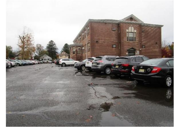
A bioretention system can be installed to capture, treat, and infiltrate roof runoff. A row of parking spaces can be replaced with pervious pavement to capture and infiltrate stormwater. A preliminary soil assessment suggests that the soils have suitable drainage characteristics for green infrastructure.
