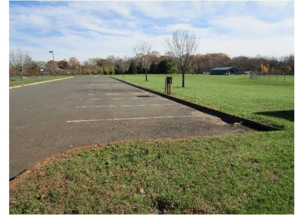
Rows of parking spaces can be replaced with pervious pavement to capture and infiltrate stormwater. A bioretention system can be installed at the front of the building to capture, treat, and infiltrate parking lot runoff via curb cuts. A preliminary soil assessment suggests that the soils have suitable drainage characteristics for green infrastructure.
