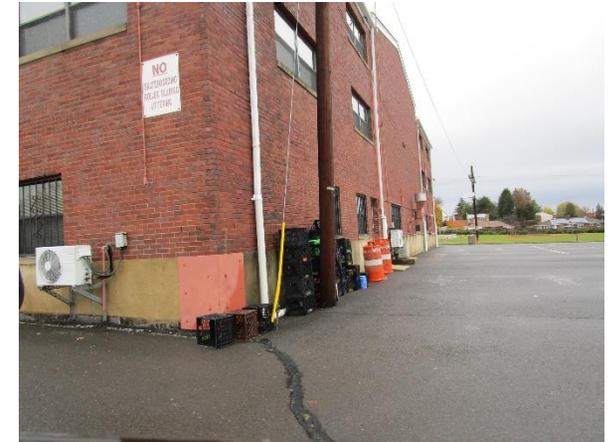
A bioretention system can be installed in front of the school to capture, treat, and infiltrate roof runoff. Parking spaces can be replaced with pervious pavement to capture and infiltrate stormwater. A preliminary soil assessment suggests that the soils have suitable drainage characteristics for green infrastructure.
