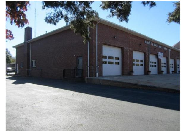
A bioretention system can be installed to capture, treat, and infiltrate runoff from the roof. Parking spaces can be replaced with pervious pavement to capture and infiltrate stormwater. Rainwater can be harvested by installing a cistern at the fire company. The water can be used for cleaning emergency vehicles or for conducting car wash fundraisers. A preliminary soil assessment suggests that the soils have suitable drainage characteristics for green infrastructure.
