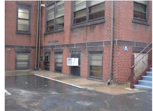
Parking spaces can be replaced with pervious pavement to capture and infiltrate stormwater. Planter boxes can be constructed to allow roof runoff to be reused. A preliminary soil assessment suggests that the soils have suitable drainage characteristics for green infrastructure.
