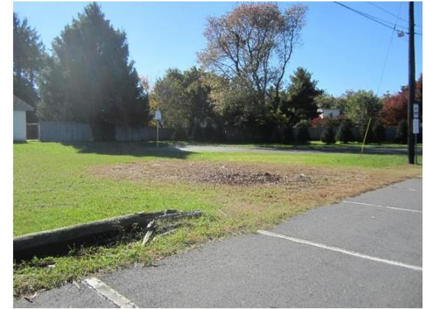
The existing swale behind the gray building at the ball field can be converted into a bioswale. Additionally, a bioretention system can be installed to capture, treat, and infiltrate parking lot runoff. A preliminary soil assessment suggests that the soils have suitable drainage characteristics for green infrastructure.
