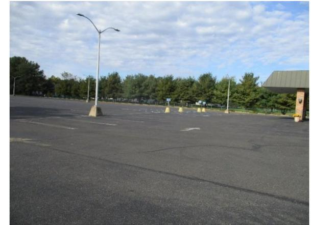
Rainwater can be harvested by installing a cistern at the fire company. The water can be used for cleaning emergency vehicles or for conducting car wash fundraisers. Parking spaces can be replaced with pervious pavement to capture and infiltrate stormwater. A preliminary soil assessment suggests that the soils have suitable drainage characteristics for green infrastructure.
