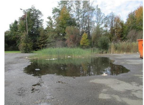
A section of the parking lot can be depaved, and a bioretention system can be installed to capture, treat, and infiltrate parking lot runoff. Parking spaces can be replaced with pervious pavement to capture and infiltrate stormwater from the parking lot and the building's rooftop. A preliminary soil assessment suggests that the soils have suitable drainage characteristics for green infrastructure.
