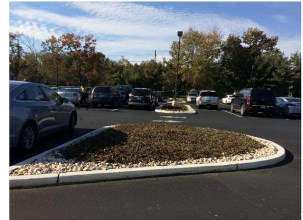
Parking spaces can be replaced with pervious pavement to capture and infiltrate stormwater. Parking lot islands can be transformed into bioretention systems to capture, treat, and infiltrate parking lot runoff. A preliminary soil assessment suggests that the soils have suitable drainage characteristics for green infrastructure.
